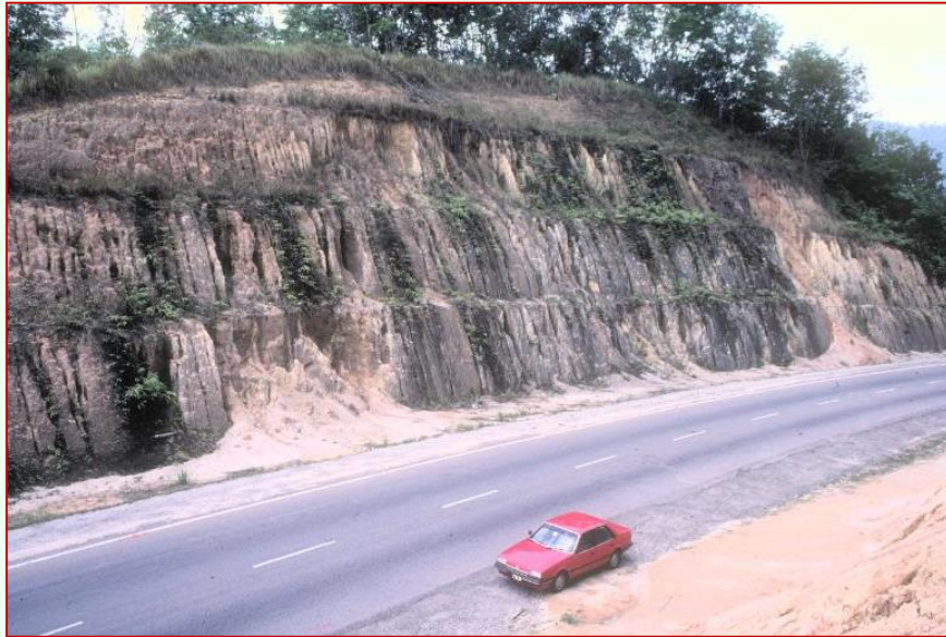
KL – Karak Highway – erosion only from direct rainfall on the face – no catchment above the face
